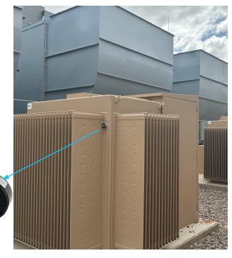
About the size of a hockey puck, the small and unobtrusive sensor adheres to crucial equipment and allows for real-time data.
